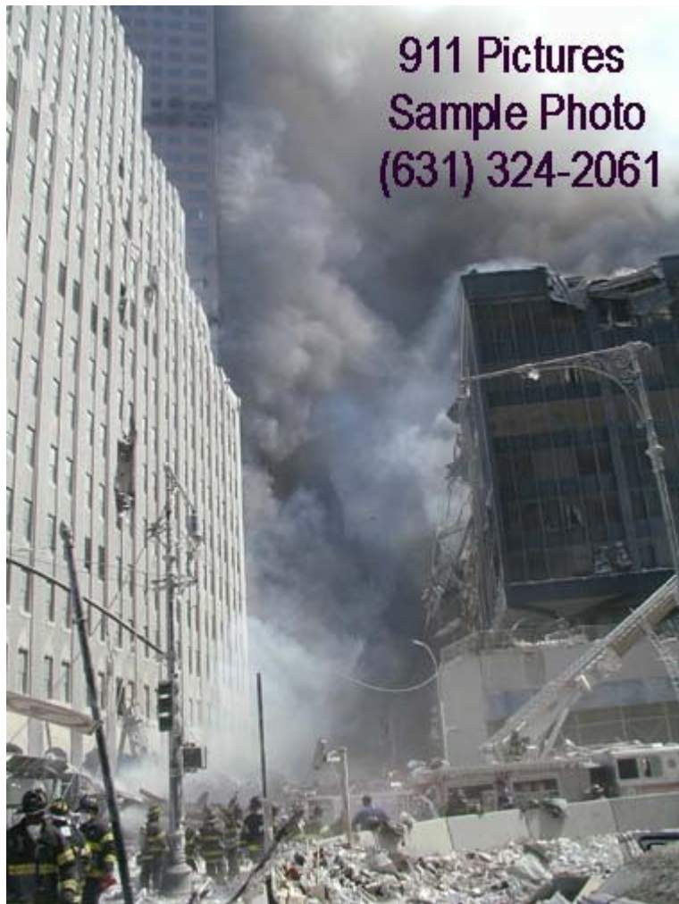
Figure Vesey1. Looking east on Vesey Street from the West Street intersection after WTC1 was destroyed, the Verizon building is on the left, WTC7 is behind the Verizon building, and WTC6 is on the right. It looks like you could drive down Vesey Street in a four-wheel Jeep. Obviously most of WTC1 didn't fall into Vesey Street. (9/11/01) Source
