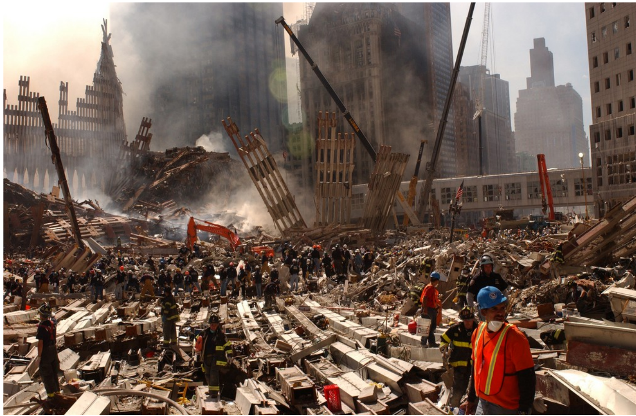
Figure 55(b). WTC3 was reduced to this 3-4 story high if narrow debris stack. A lower section of WTC1's west wall lays across the West Side Highway.
