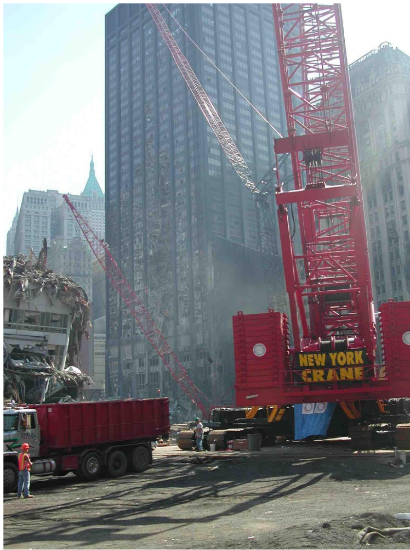
Figure 27. Note that solid debris appears to have hit only the lower half of this 40-story building (Bankers Trust). However, the top few floors appear to have had their windows blown out.
