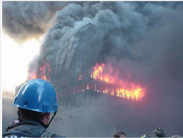
Figure 13(a). close up building ablaze Maybe they set WTC5 on fire for a "smokescreen" after the fact? Why would this building be on fire so viscously and so FAST?
