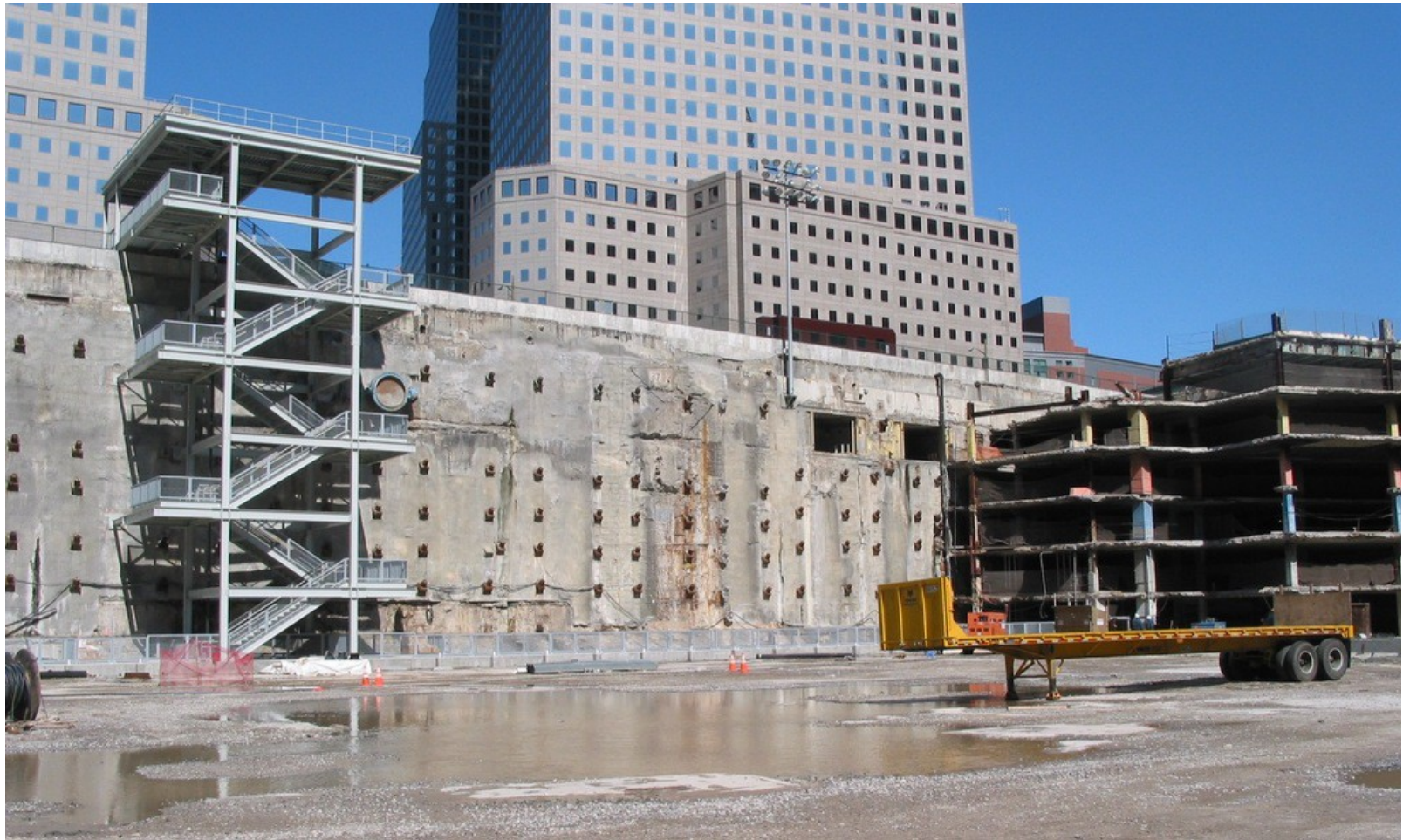
Figure 101. But, clearly the bathtub survived. This is a view from the footprint of WTC1. Notice the parking structure that was under WTC6 survived.
