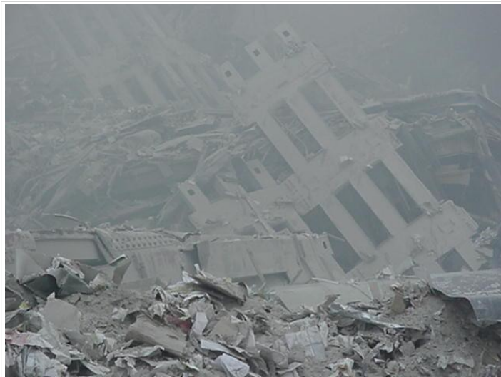
Figure 16(a). rubble close up
