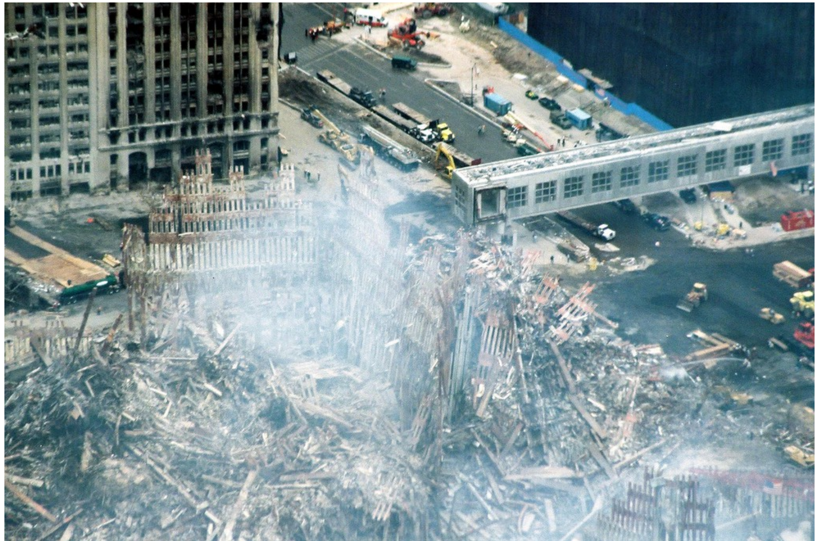
Figure 313. Most of WTC3 disappeared during the destruction of WTC1. The pedestrian walkway over the West Side Highway was connected to something that is no longer there. The remains of WTC2 can be seen near the center of the photo and the remains of WTC1 are partly visible in the lower right corner.
