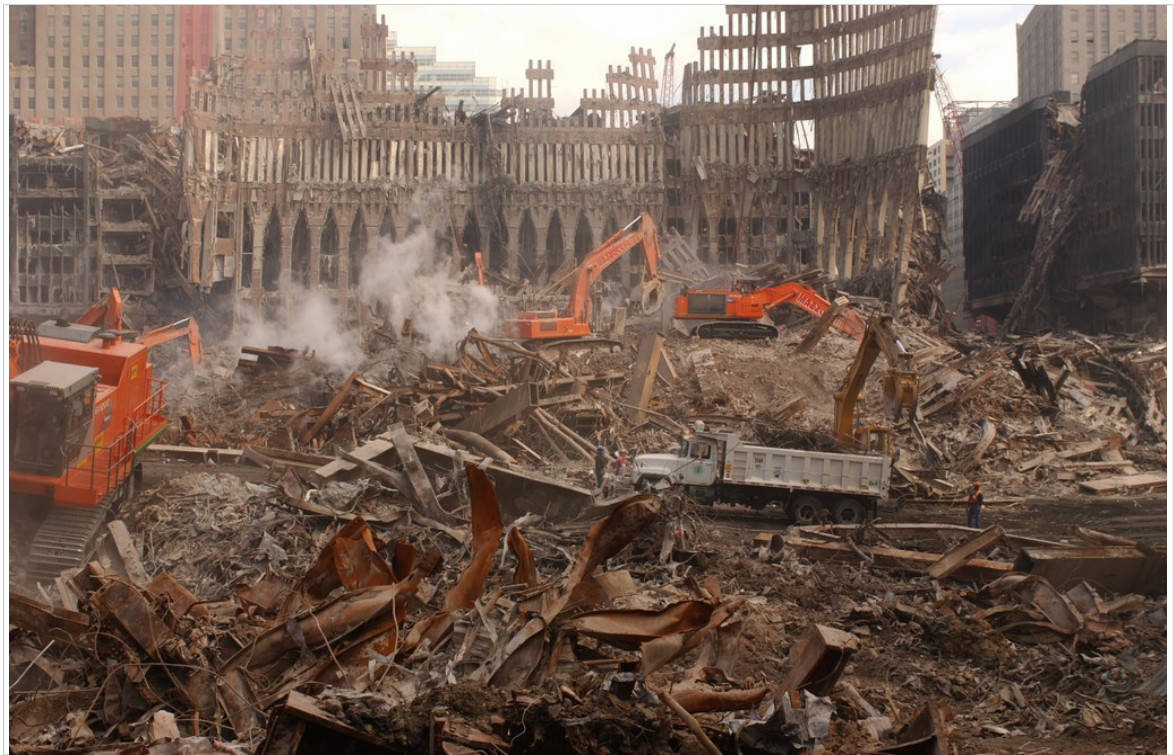
Figure lobby(b). The lobby of WTC1 after 9/11. (9/??/01) Source
