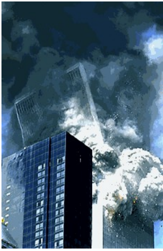
Figure 74(d). Demolition starts bad: the top 300 feet of WTC 2 tilted as much as 23° before being Blown to Kingdom Come .
