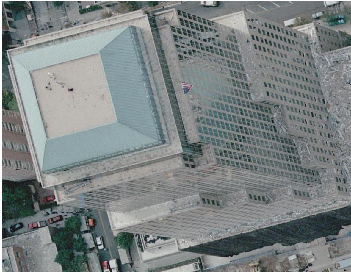
Figure 10. WFC2 had only pulverized dust and WTC aluminum cladding on its roofs. WFC2 suffered only window damage only to its lower floors, despite the destruction of a 1/4-mile high building across the street.
