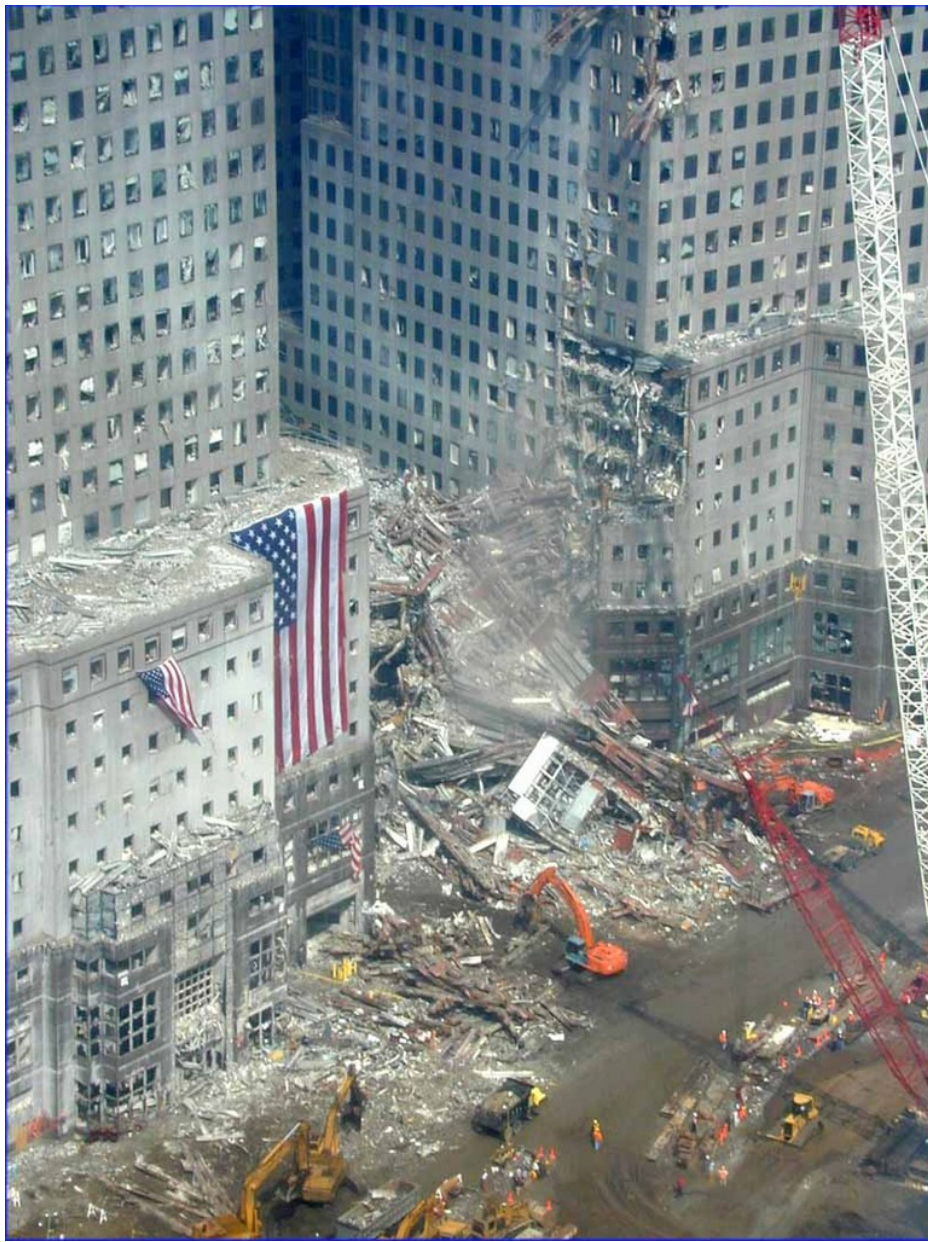
Figure 29. Note the blown out windows at the WFC. There appears to be no other damage to the façade of WFC2 on left.
