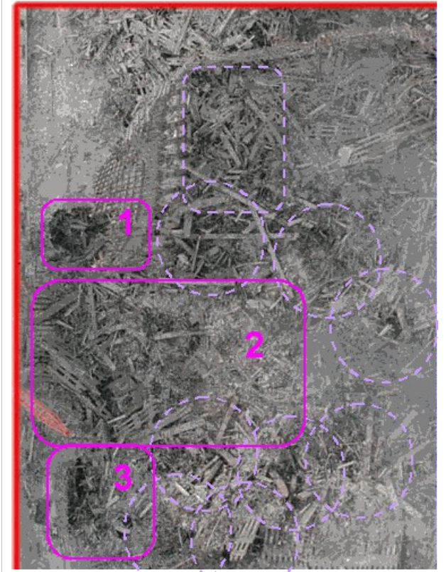
Figure 302(b). Figure 302 is located in zone 2, above. Overhanging debris was removed before ladder was lowered into hole 2.
