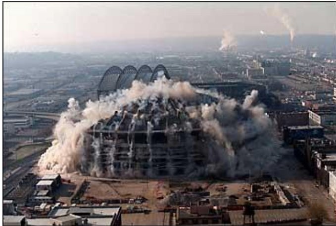
(c) The right and left sides are "pulled" first to fold the building inward.
