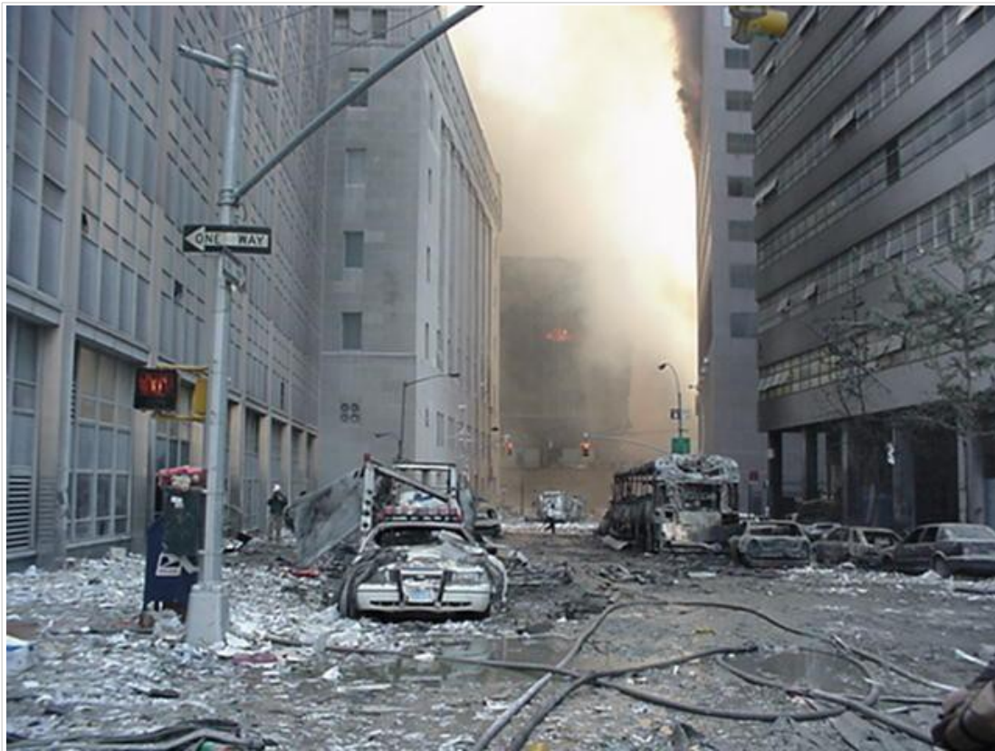
Figure 9(a). block with fire at end
