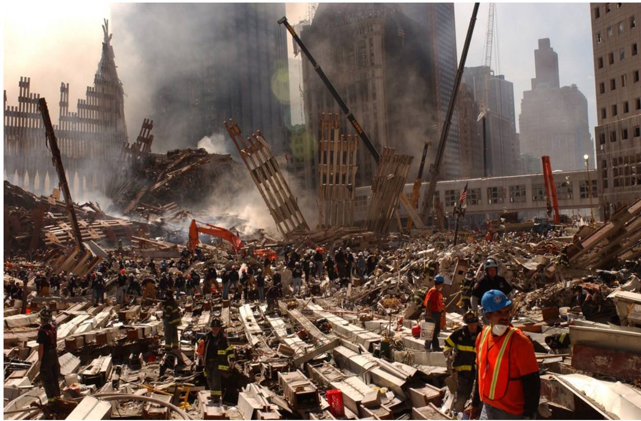
Figure 55(b). The remarkable "lay down" of steel wheatchex from the lower stories of WTC1 on West Street (West Side Highway). The WTC3 debris pile is in the background, next to the unsupported WTC2 wall. (9/13/01) Source
