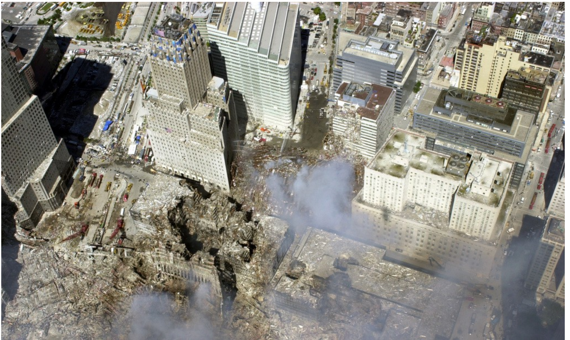
Figure 56. This photo highlights the depth of the hole in WTC6. The "smoke" or pulverized dust from debris appears to have diminished in comparison to Figure 55(a). While there is abundance of aluminum cladding on the roofs of buildings 5 and 6, there is little or none in the holes.
