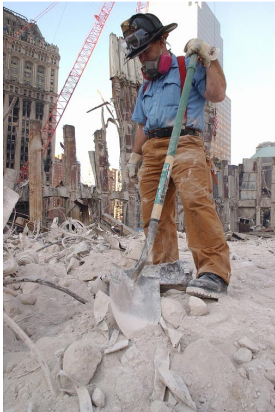
Figure 84(a). Scooping up the building.
