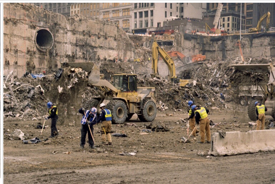
Figure 308. The southeast corner of the big bathtub again. Dust or smoke rises from the pile. The workers are wearing respirators, not simple dust masks, six months after 9/11. The dust or haze is very fine and does not settle out like regular dust would behind a vehicle on a dirt road. The policemen apparently are sifting through debris, looking for body parts (photo filed 3/15/02) Source
