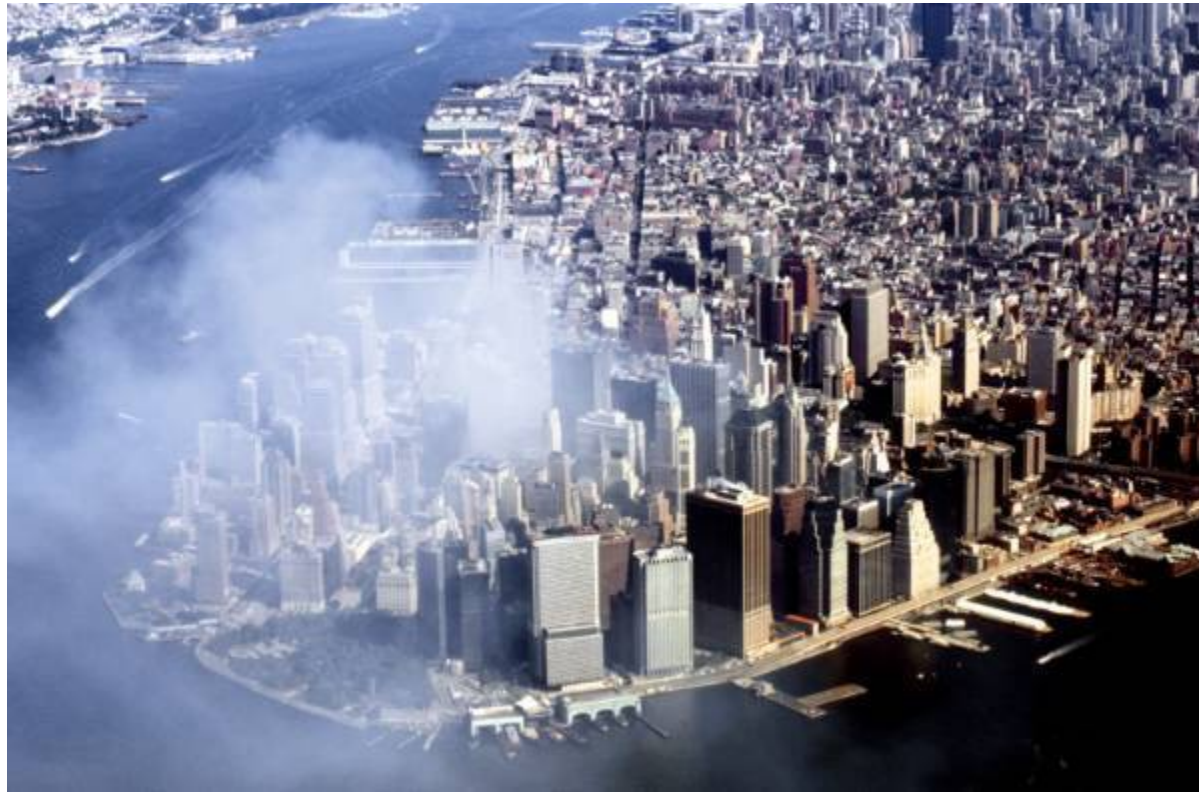
Figure 41a. "Fumes" from the site were visible for days.
