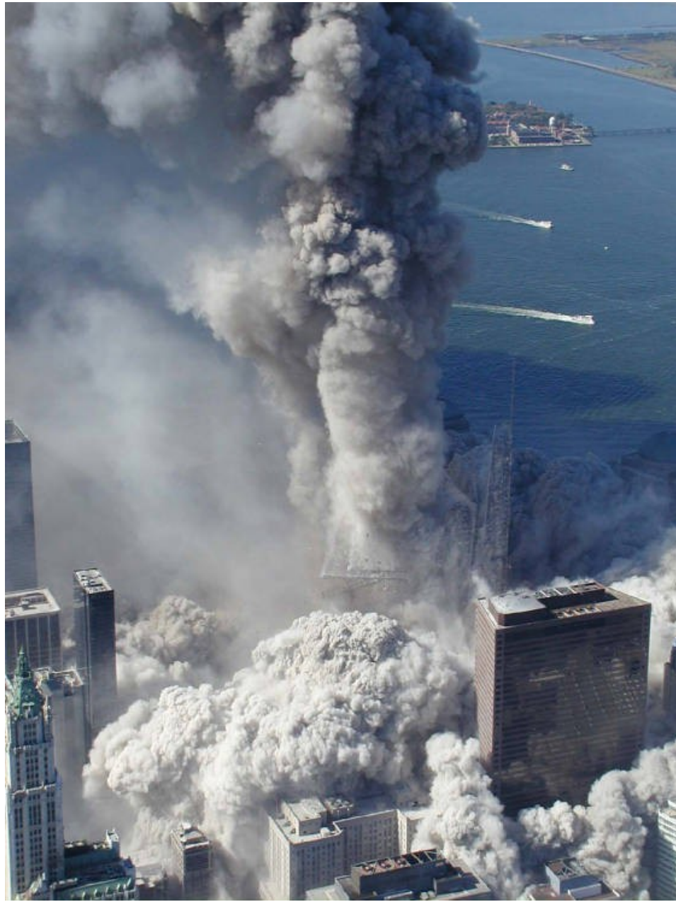
Figure 34. Building turns to dust.
