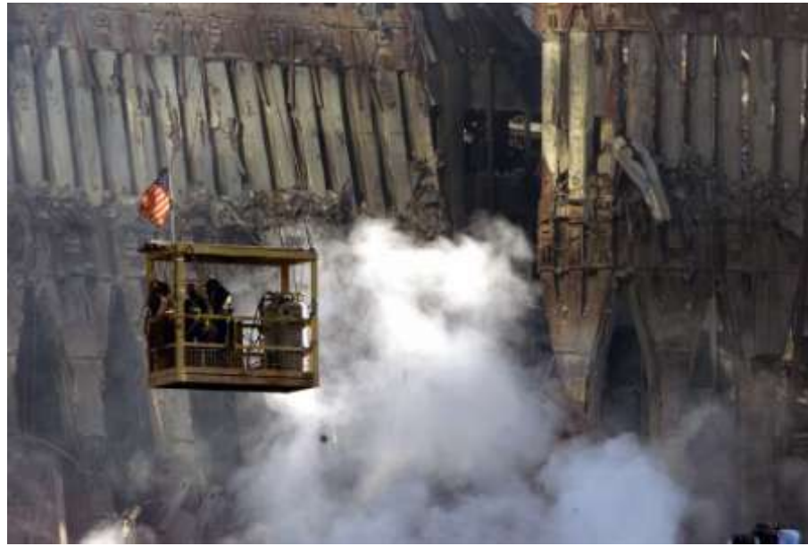
Figure 81. These look like healthy beams, not damaged/failed beams. These folks are suspended only a few stories above the ground. (little to no rubble pile below them)
