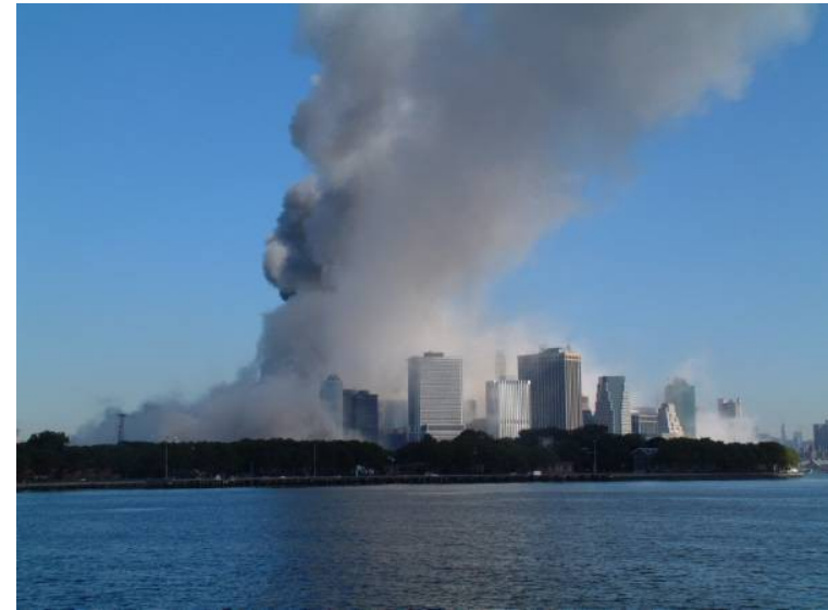
Figure 50. Ground-level view of the enormous quantity of dust wafting skyward. Conventional demolition dust does not do this.
