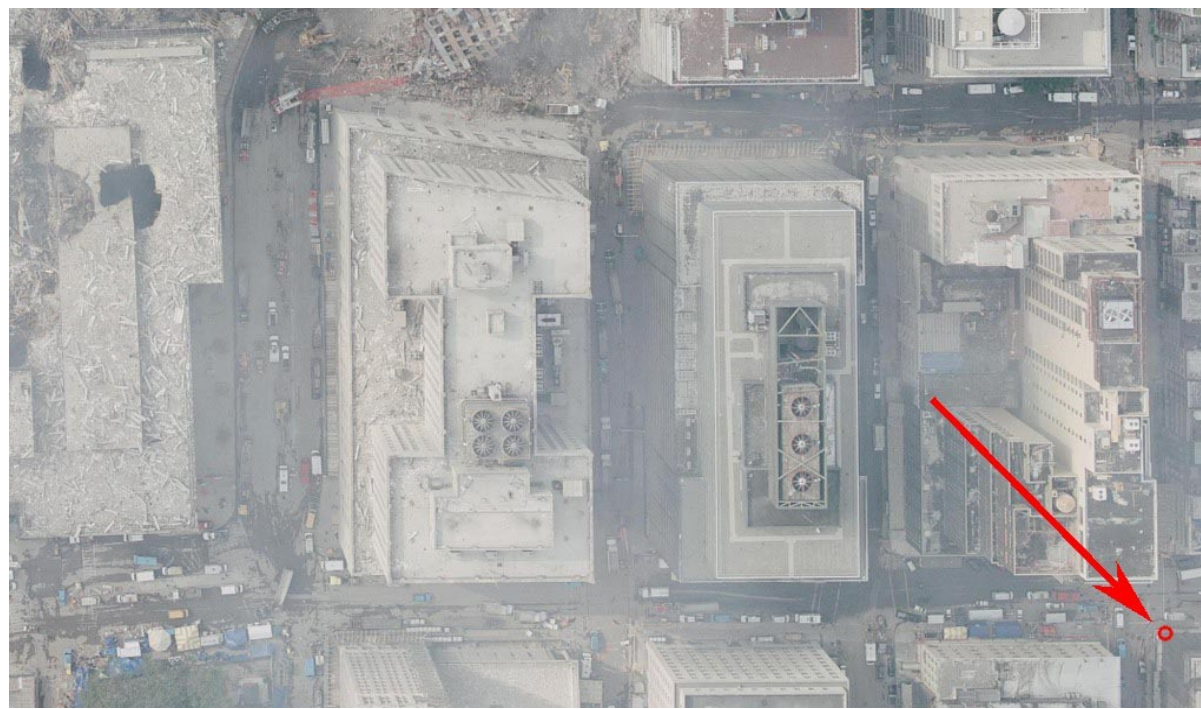
Figure 9(a). WTC5 on the left, the U.S. Postal Service building, and the two buildings to the right (north) of the postal building, have only modest dust and a few pieces of aluminum cladding on their roofs. A jet engine piece was found at the corner of Murray and Church Streets as indicated in Figure 9.
