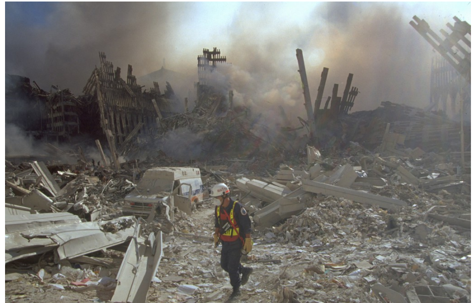
Figure 87(e). The "rubble pile" from WTC1 is essentially non-existent. The ambulance is parked at ground level in front of WTC1. WTC6, which had been an eight-story building, towers over the remains of WTC1.
