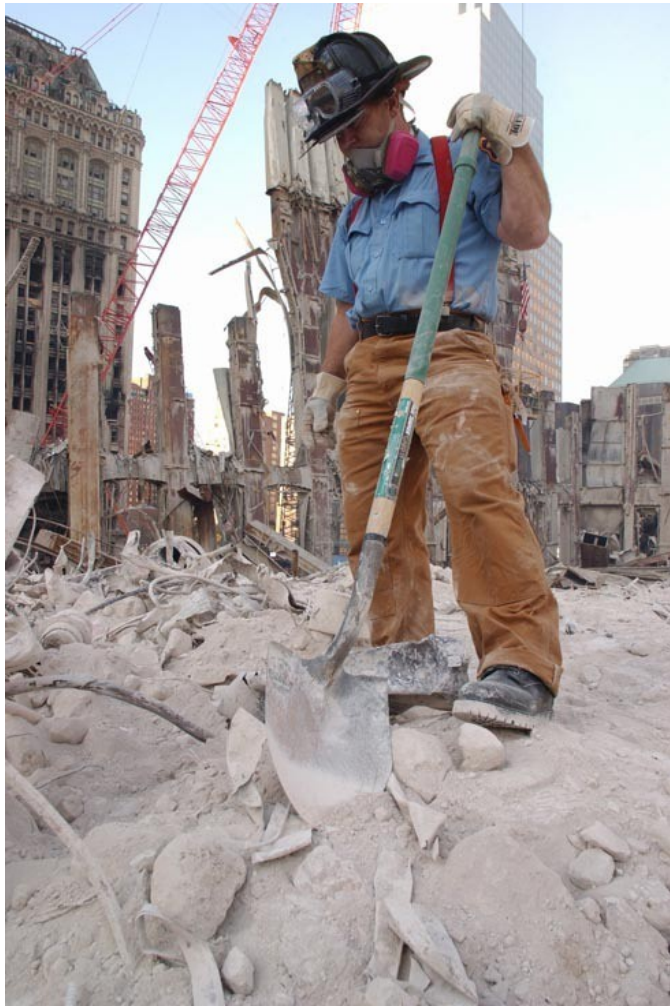
Figure 46. Scooping up the building.
