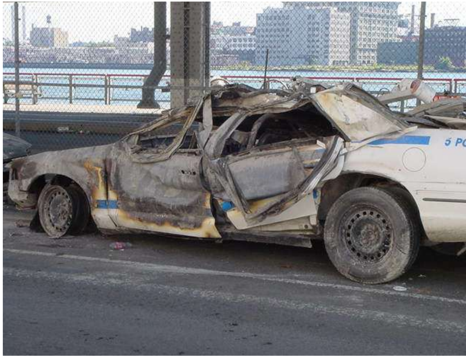
Figure 64. Peculiar wilting of car doors and deformed window surrounds on FDR Drive.
