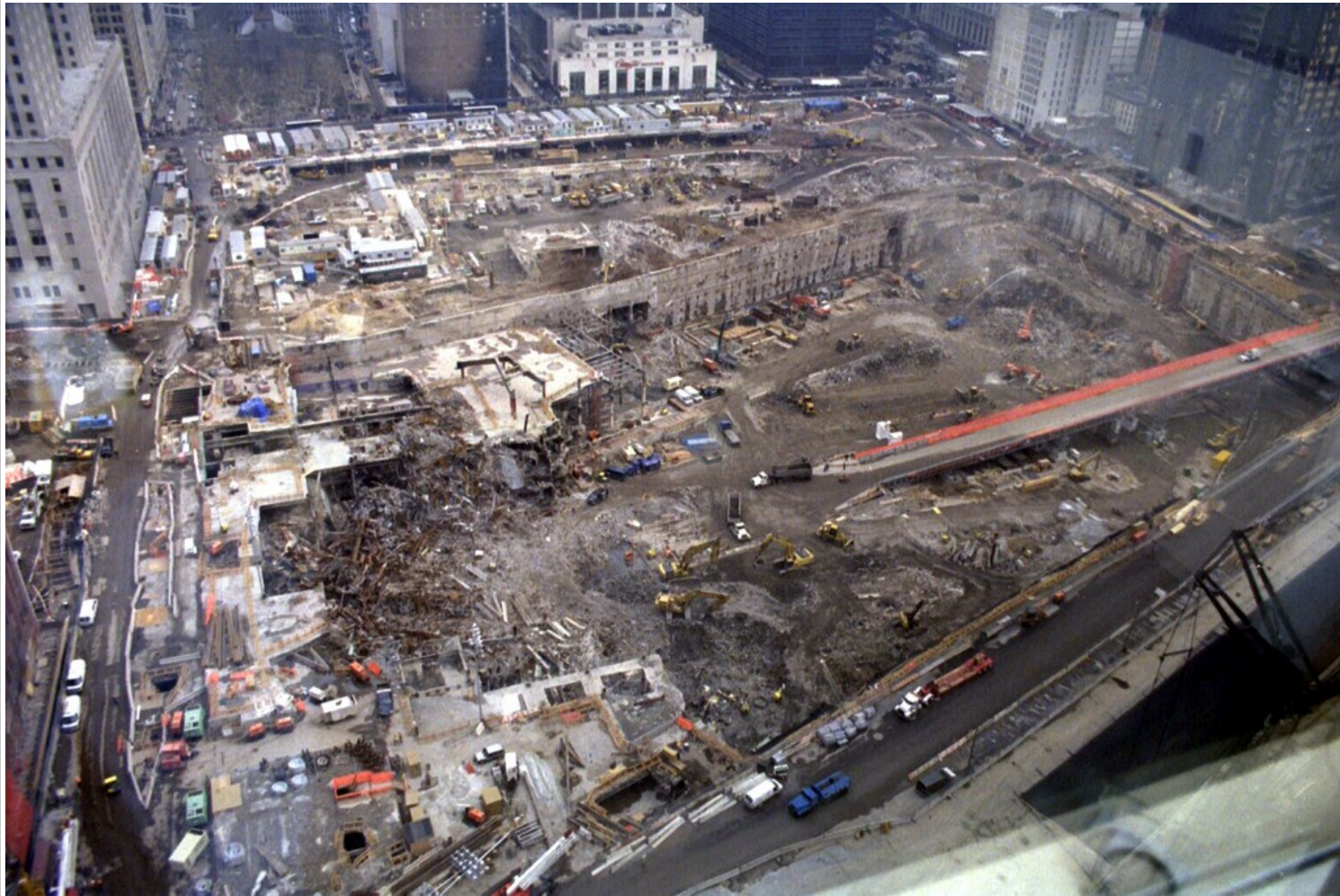
Figure 15. (old Figure 9.) The nearly cleaned-out bathtub. (March 15, 2002)
