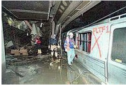
Figure 6. (old Figure 2.) WTC Station Platform after the event; this PATH train wasn't crushed.
