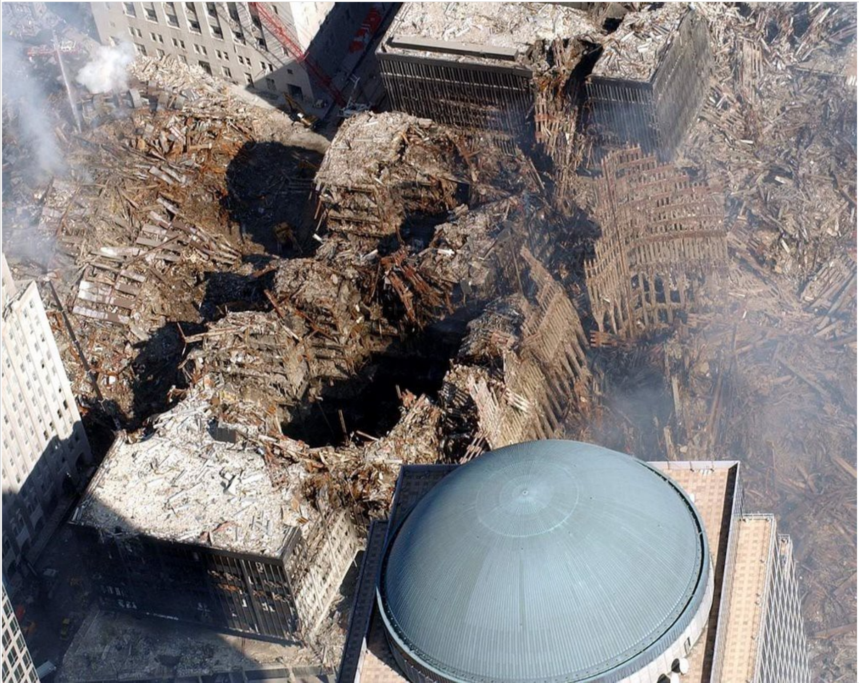
Figure 57(b). A view over the dome of WFC2 shows the damage to WTC6 in the center of the photo. To the left is the
